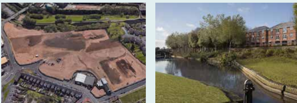
Galton Lock; a £32m development consisting of 180 two, three and four-bedroom new homes off Mafeking Road and Lewisham Road, Smethwick.
